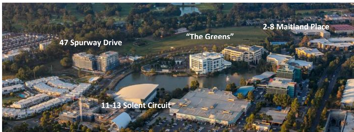
Image 3: Oblique Aerial view of site showing Norwest Markettown and Metro Station in foreground.
